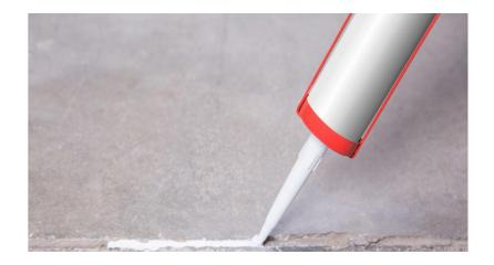
Based on polyurethane resins and other additives to fill expansion joints that are in transit.
