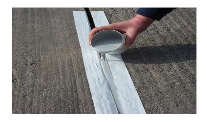
It is a two-component hot-water mastic based on tar and polymer, which, while possessing elasticity, is quite resistant to a variety of solvents and petroleum products, gasoline and fuel.
